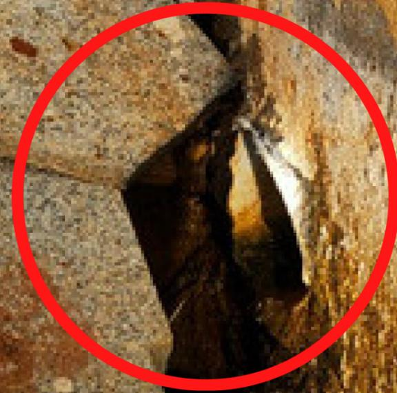
**Water leaking in Basement : spalling**
