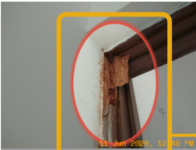
Termite attack on door frame
